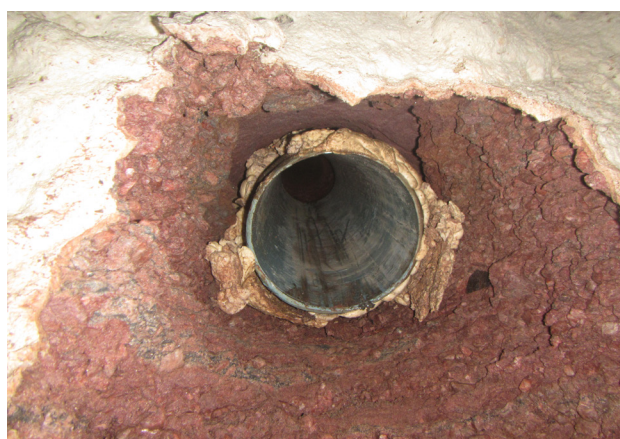
Once the holes had been drilled, casings were installed in order to prevent the holes from collapsing due to the soft formations
