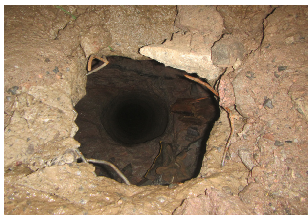
Once the holes had been drilled, casings were installed in order to prevent the holes from collapsing due to the soft formations
