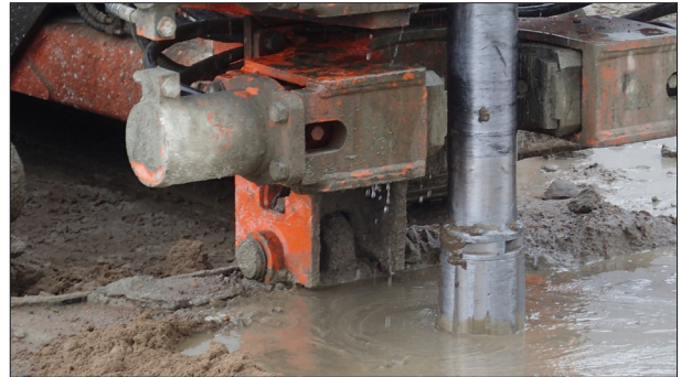
Jet grouting in progress
