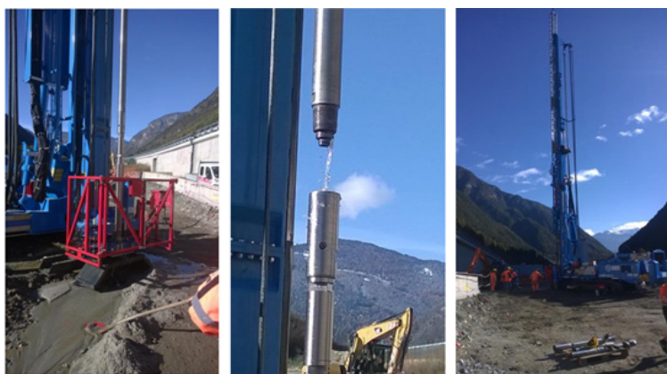
Left: W120 Hammer and monitor, Middle: Monitor and triple fluid rods, Right: Solimec SM 28 in action
