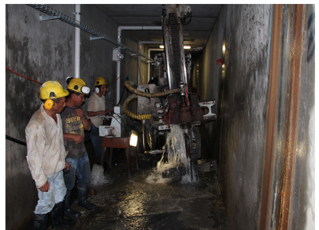
Drilling in action in one of the galleries
