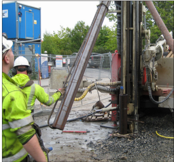
Another casing with drill rod is added to the drill string
