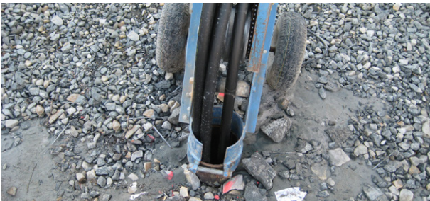
Installing the geothermal cables
