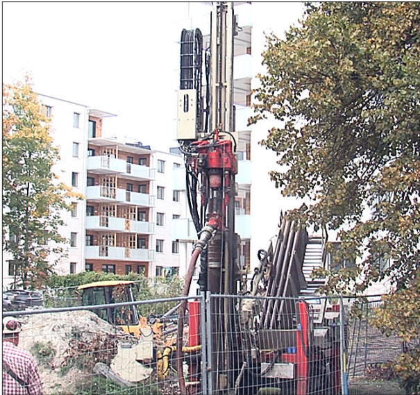
Drilling takes place close to a block of flats
