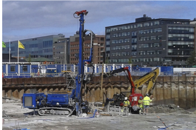
The Hütte drill rig with Wassara for Malmö Live
