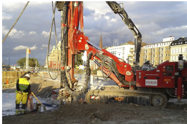
The MTD drill rig, also equipped with Wassara
