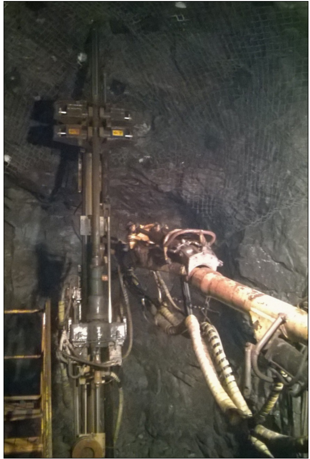
Drilling in action
