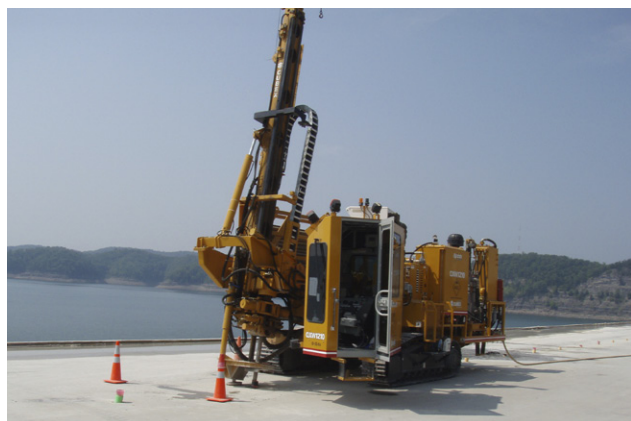
Series of Ø 95 mm (4") holes being drilled with the W80 hammer
