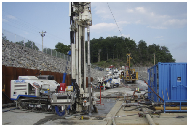
The W150 hammer, about to drill an Ø 200 mm (8") pilot hole
