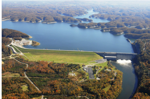
The Wolf Creek dam (Photo by Courtesy Asset, U.S. Army Corps of Engineers)
