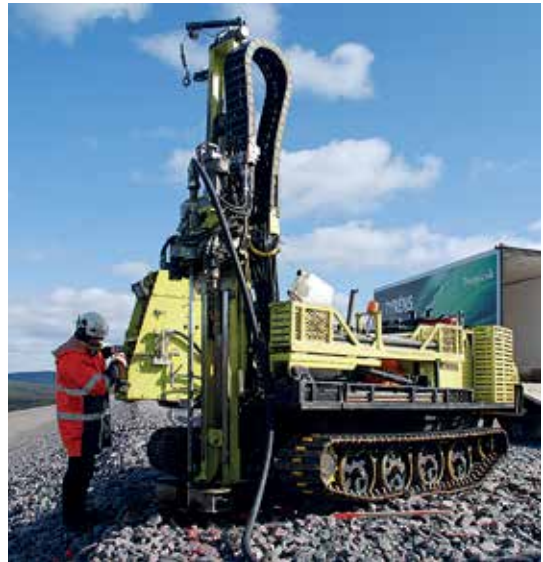
The Wassara way of installing an instrumentation casing
